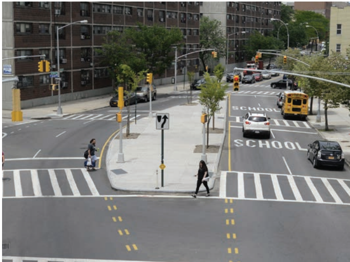
Concrete median and curb extensions
