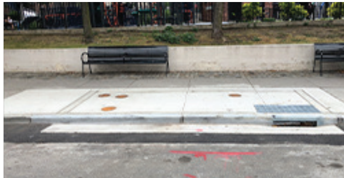
Concrete top infiltration basin
