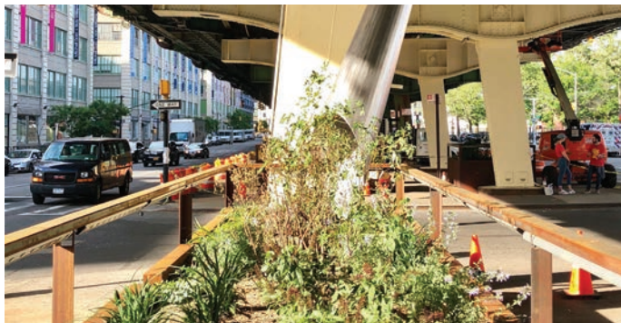
Cone-like downspouts capture storm water from the BQE elevated structures (El-Space Pilot in Sunset Park, Brooklyn)
