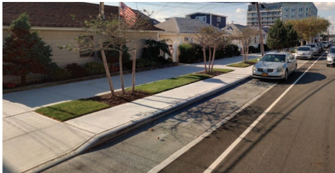
Porous concrete in the parking lane on Beach 108th St. (Rockaway Beach, Queens)
