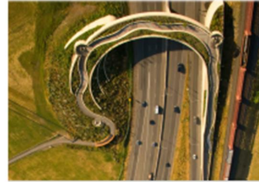
Vancouver Land Bridge (Vancouver, Canada) An earth-covered pedestrian bridge linking trail to parkland and waterfront
